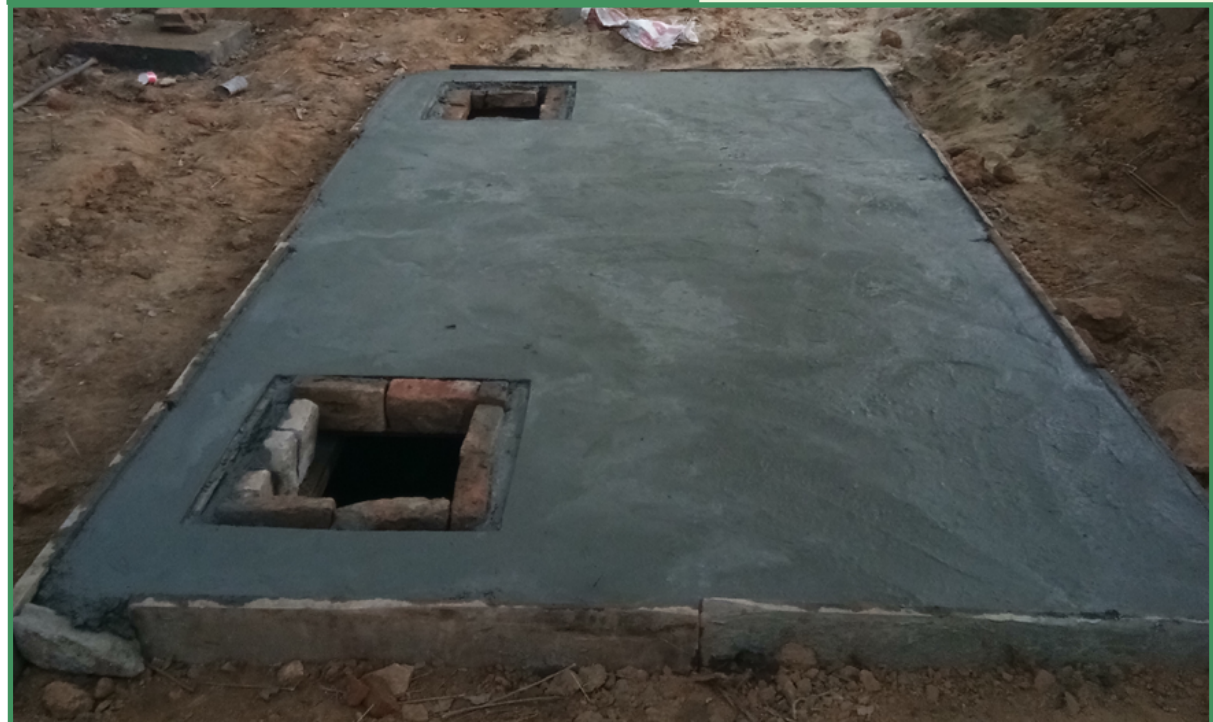
Construction of desiltation chamber for RWH
