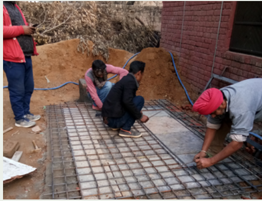
Construction of rooftop rainwater harvesting structure under progress
