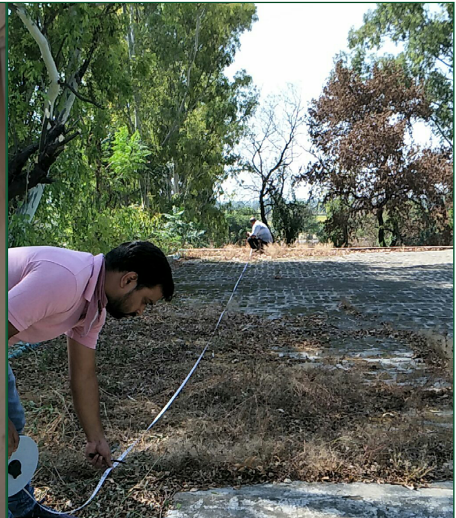
RWH measurement for roof catchment area'
