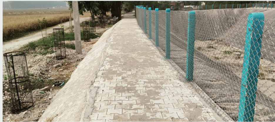
Hawas pond site after completion
