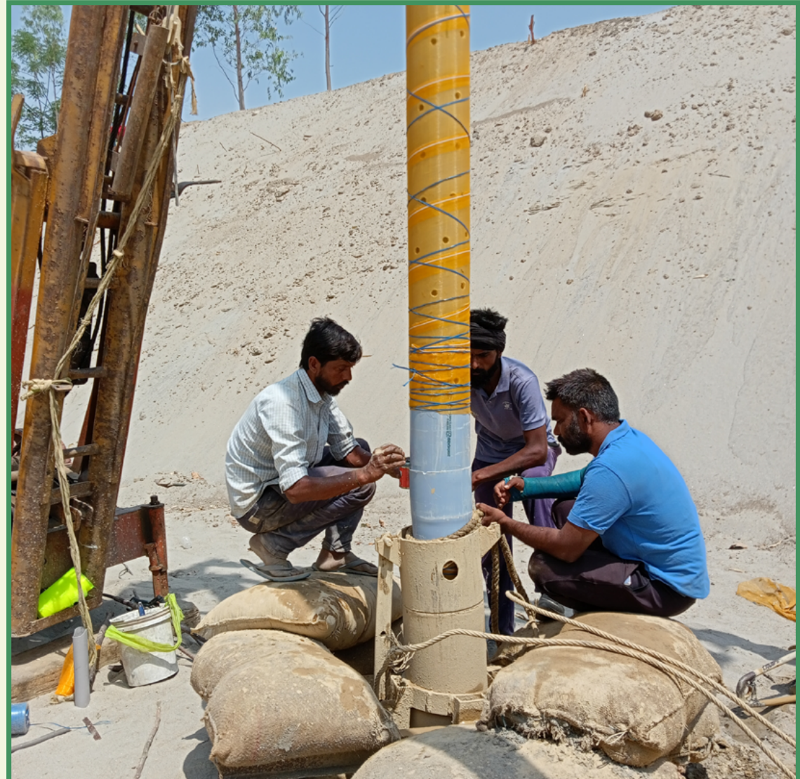
Drilling work in progress at Hawas pond site
